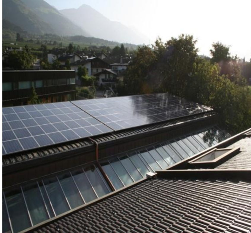
Shading problems due to nearby object / bad planning
